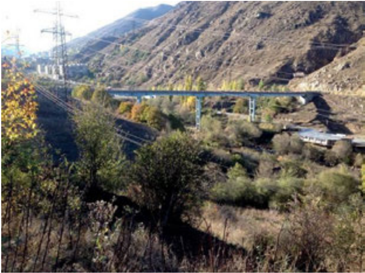
Image 124. Kajaran community. Area of the ruined cemetery existing at pk 64.0+00
