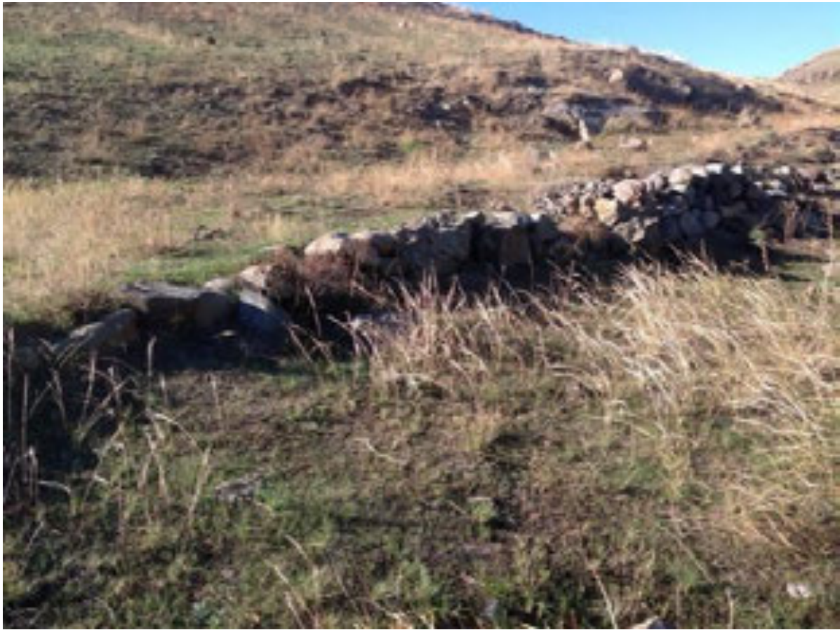
Image 37. Noravan community. Section of preserved wall at the truncated settlement recorded at pk 9.5+00
