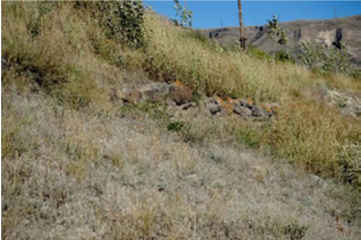
Image 43. Vaghatin community. Wall structure preserved in the area of old gardens recorded at pk 12.1+00
