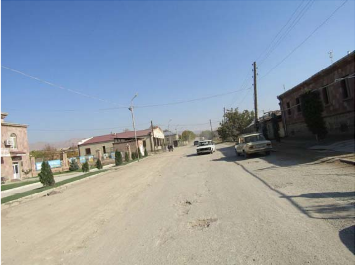
Deteriorated a/c pavement with potholes
