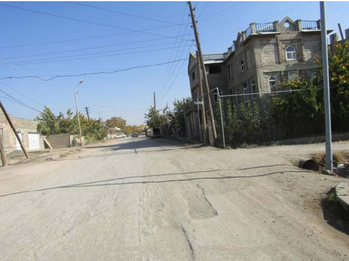
Deteriorated a/c pavement with potholes
