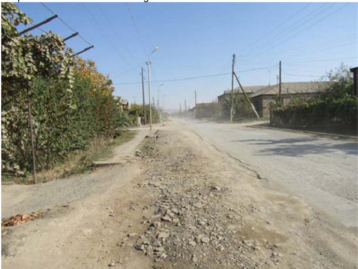
A/c pavement with cracks and edge breaks
