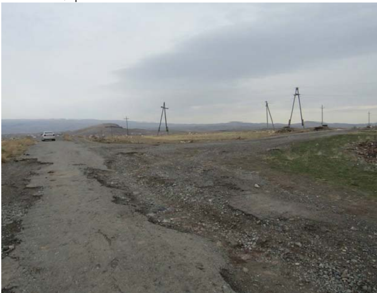
Deteriorated a/c pavement
