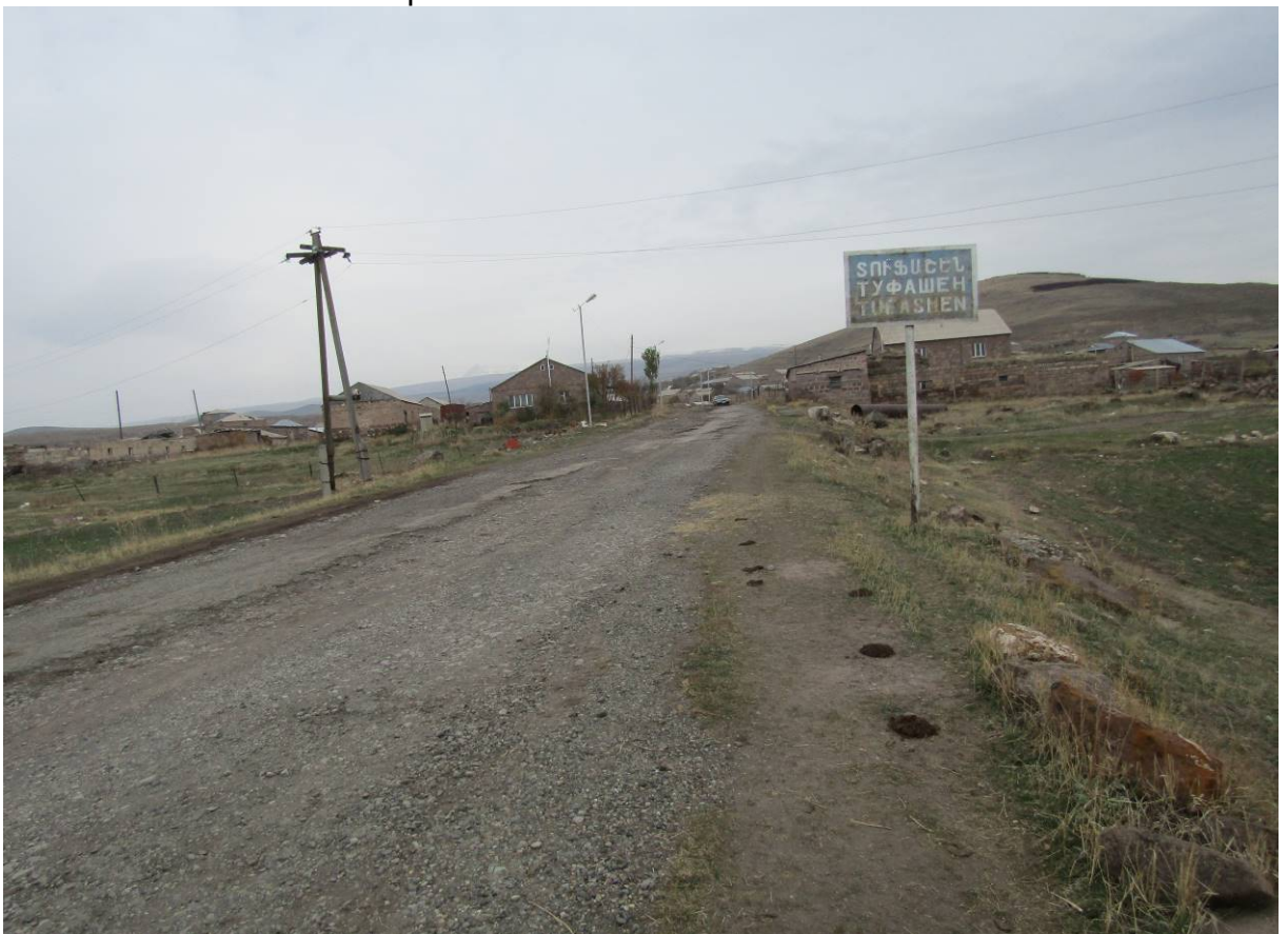
Road with deteriorated a/c pavement in Tufashen
