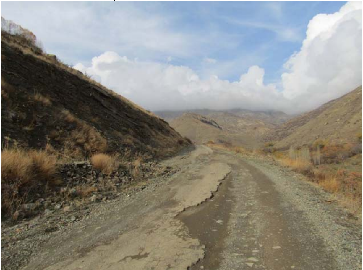
Road with deteriorated a/c pavement
