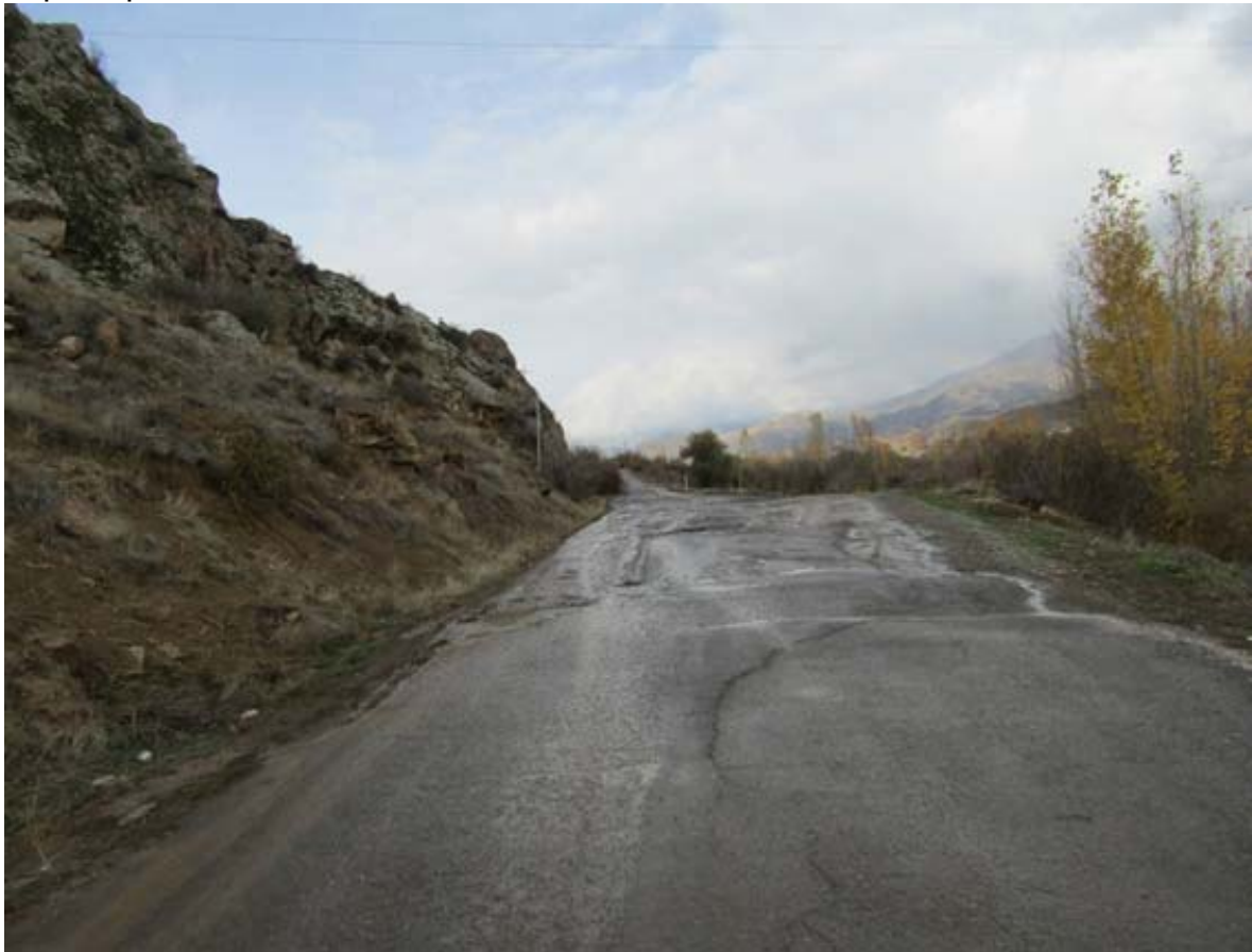
Deteriorated a/c pavement with potholes and puddles in Getap
