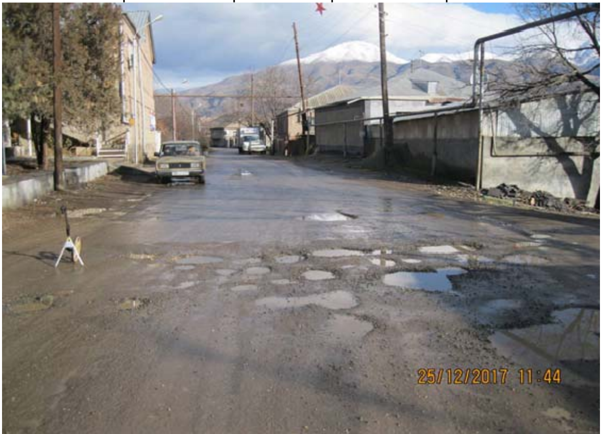
Deteriorated a/c pavement with potholes and puddles in Getap
