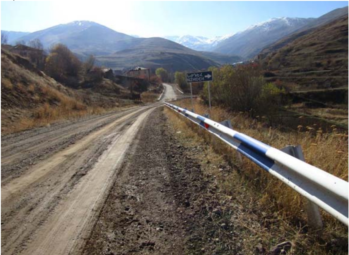
Unpaved earth road with potholes and puddles at km 4+300 in Nzhdeh community
