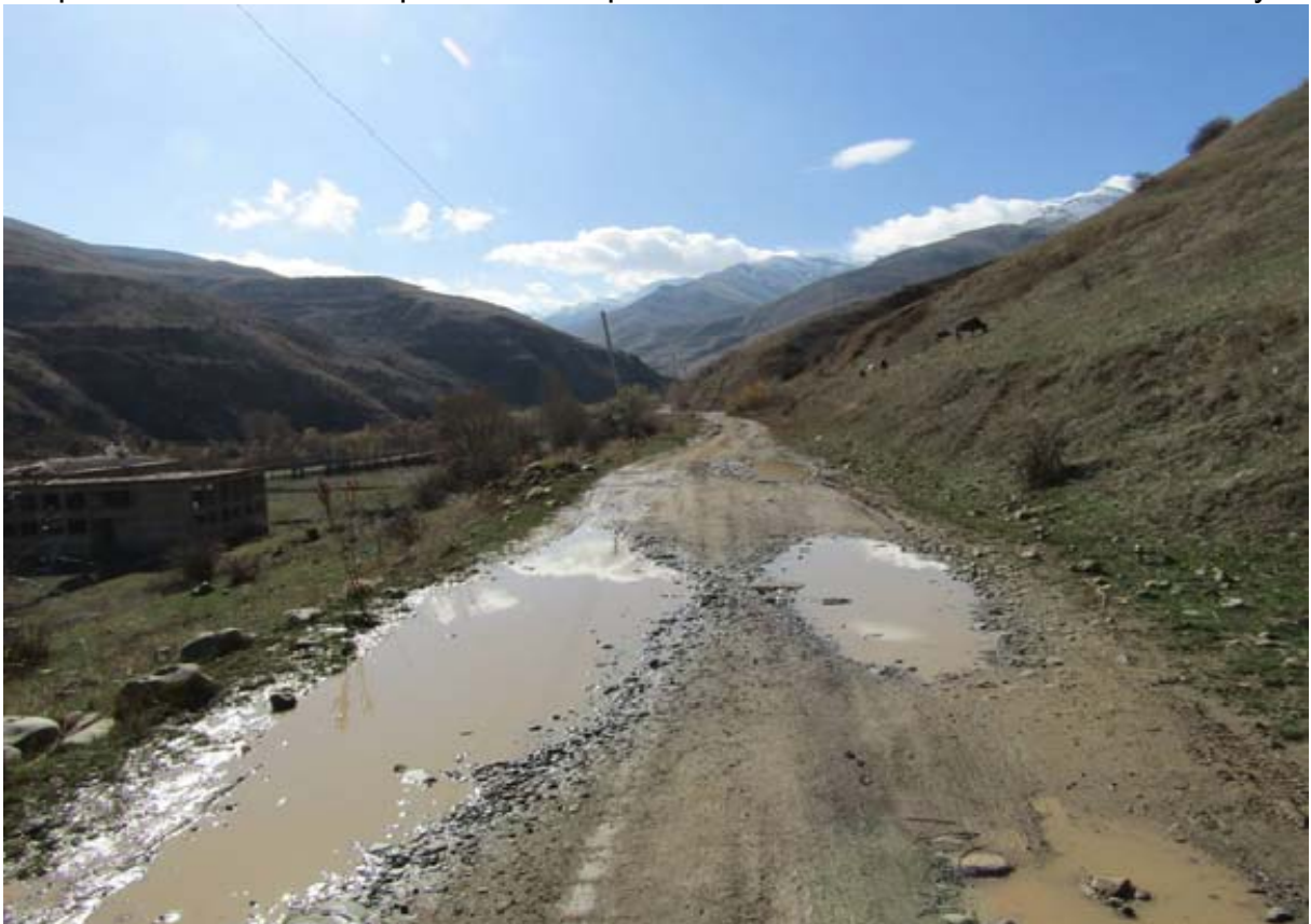
Unpaved earth road with potholes and puddles at km 4+300 in Nzhdeh community
