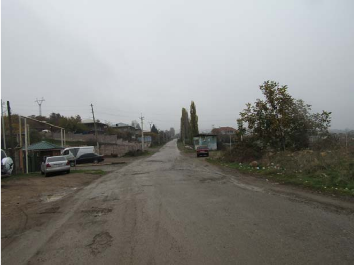
Deteriorated a/c pavement at km 1+200-km 1+250 in Getahovit community
