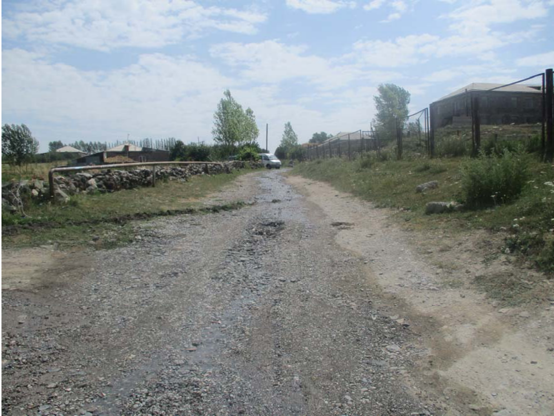
Deteriorated a/c pavement with some spots of asphalt
