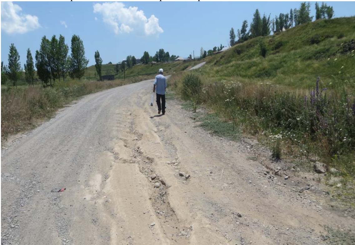
Deteriorated a/c pavement with some spots of asphalt
