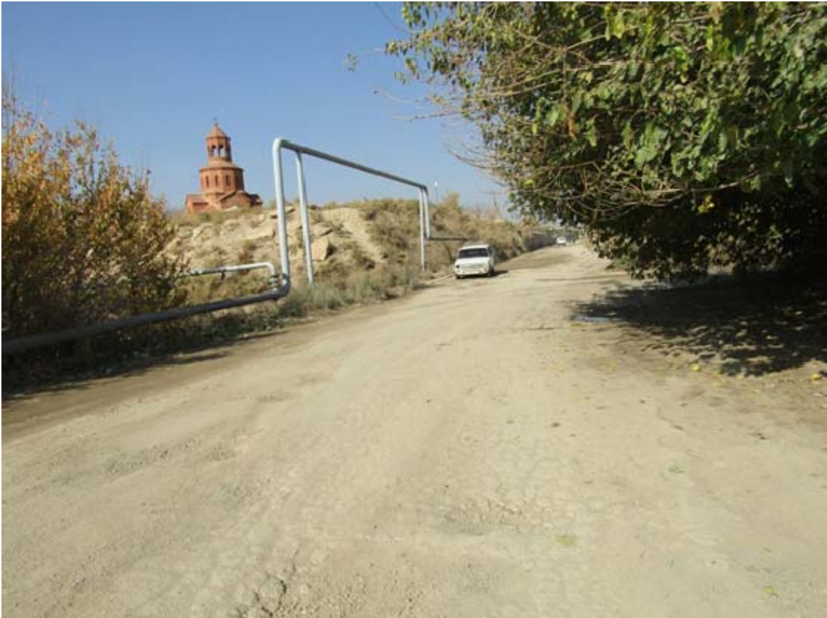
Deteriorated a/c pavement
