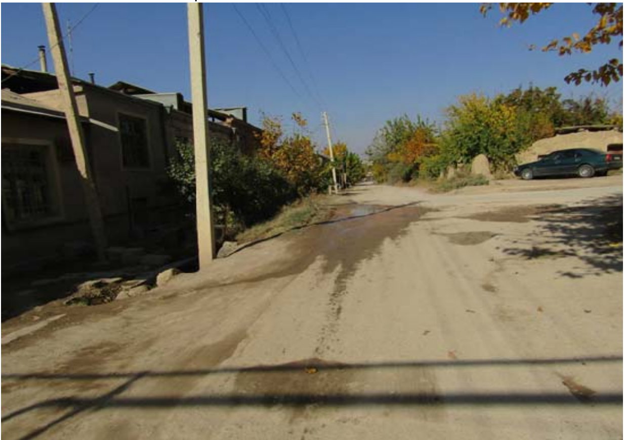
Road with deteriorated a/c pavement in Verin Artashat
