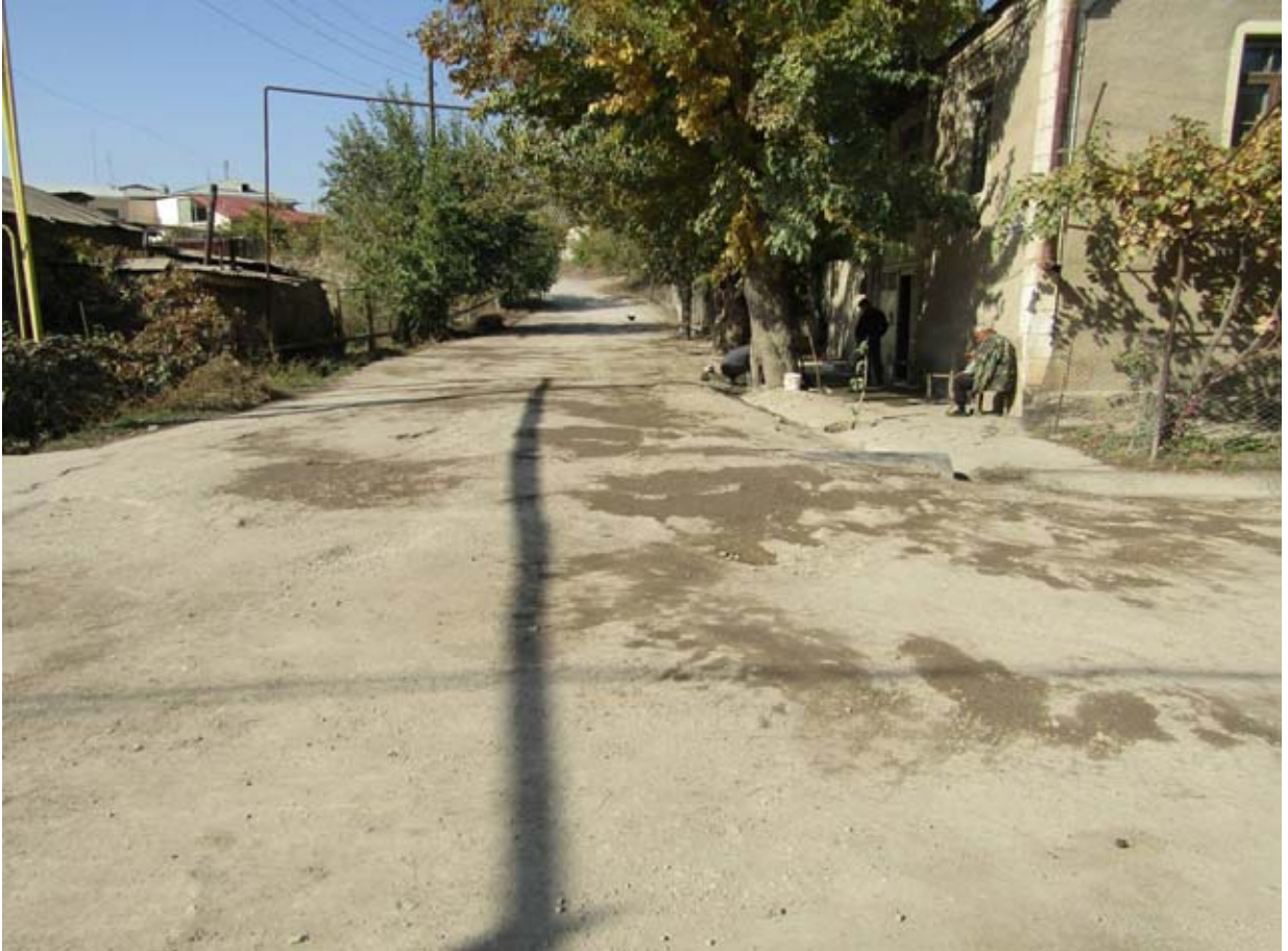
Deteriorated a/c pavement at the end of Verin Artashat
