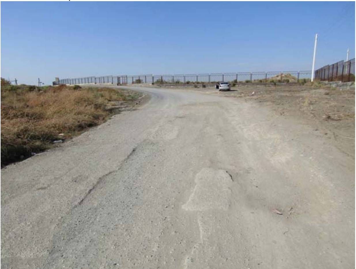
Deteriorated a/c pavement at the end of Verin Artashat
