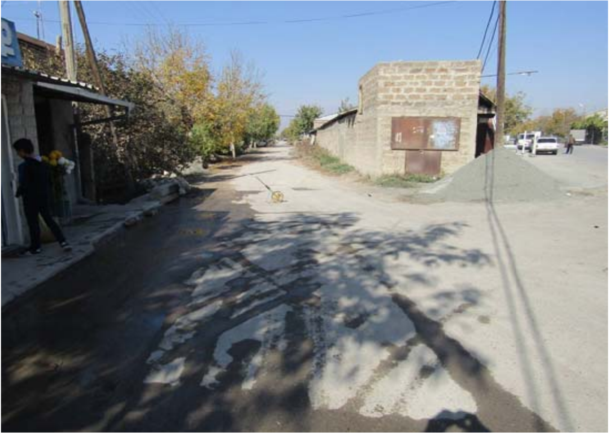
Road with deteriorated a/c pavement in Verin Artashat
