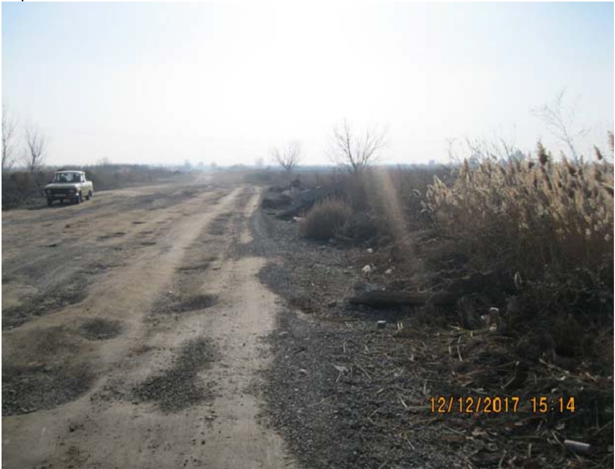
Deteriorated a/c pavement with potholes
