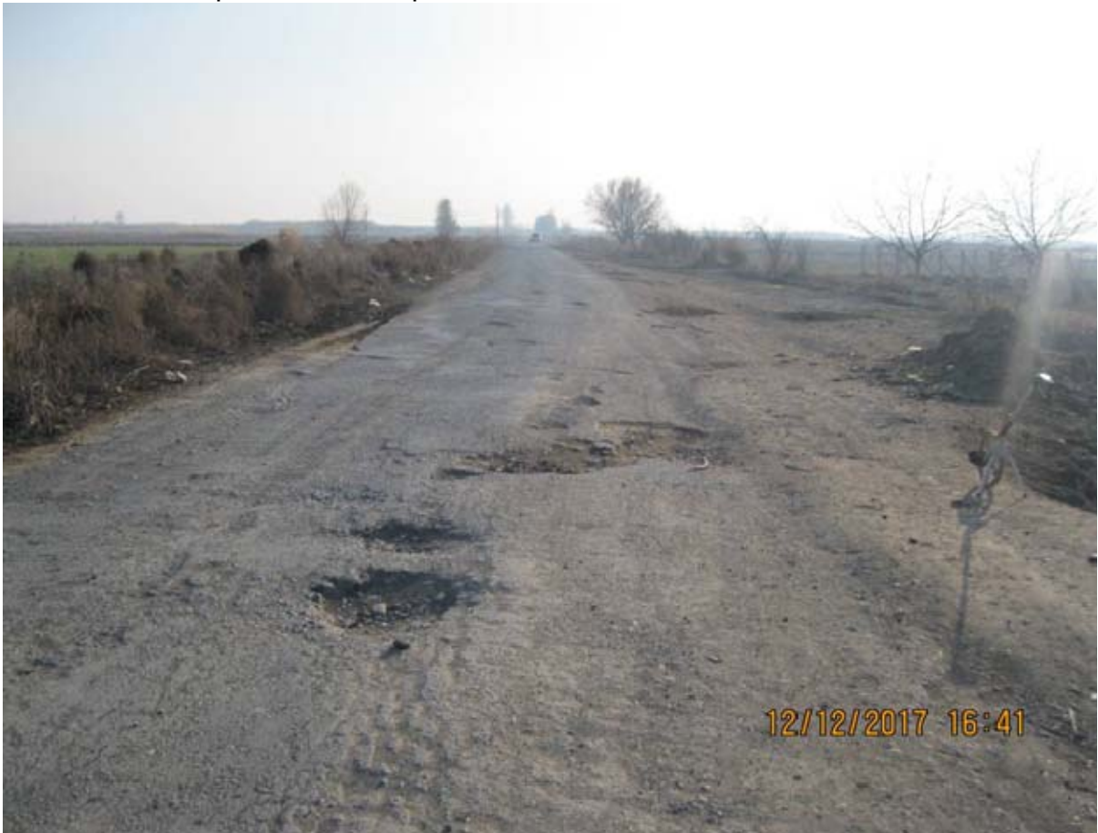
Deteriorated a/c pavement with potholes
