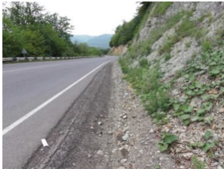
Figure 24: Road bed of Highway M6
