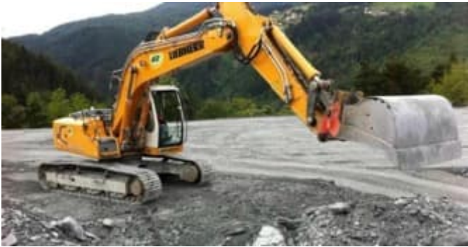
Figure 6: Excavator with attached slope-work bucket in operation
