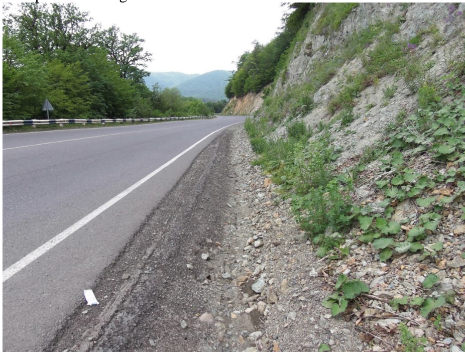
Fig. 10. Road bed of Highway M6
