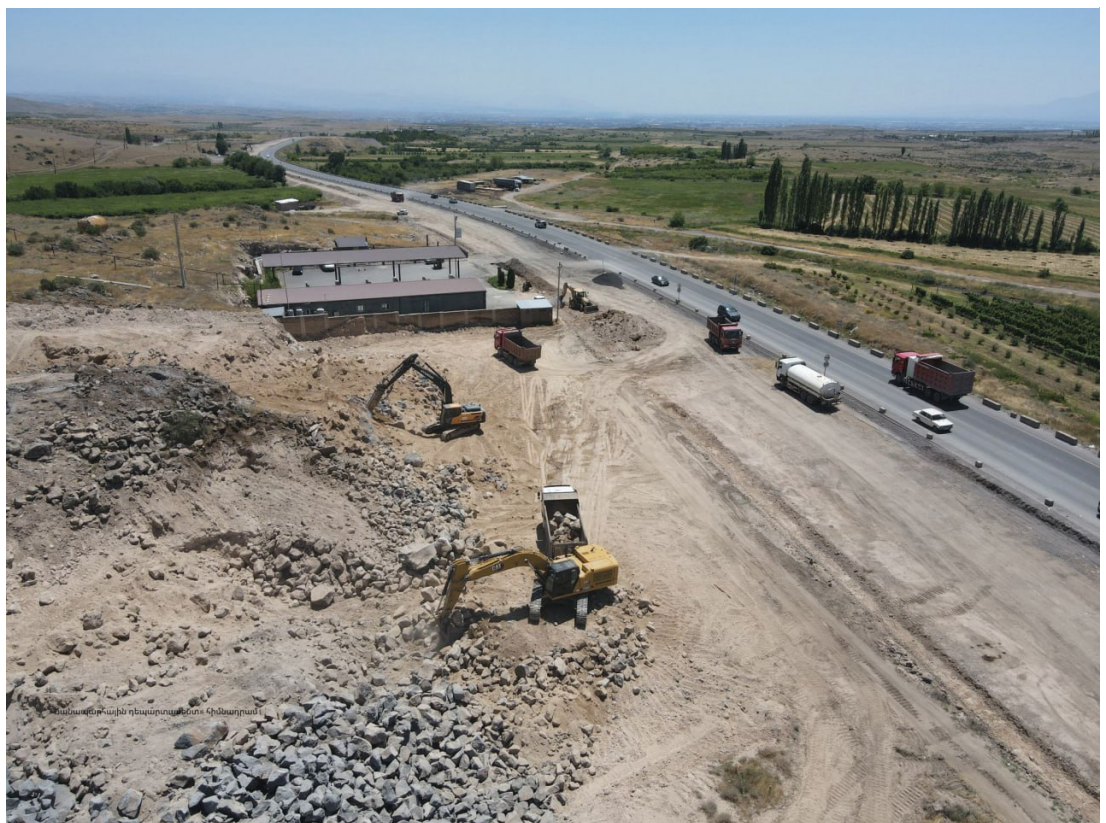
Figure 4. June 25, 2025 – km 42+900-43+000: Ongoing construction works for Task 2
