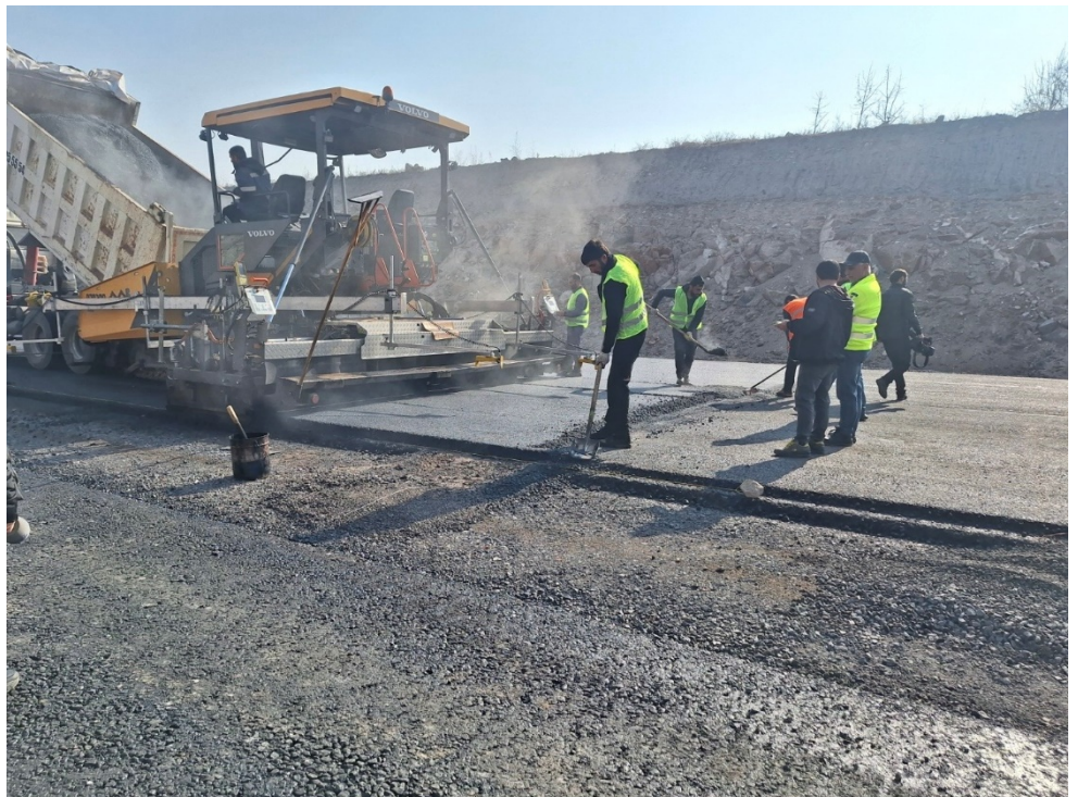
Figure 2. March 14, 2025 – km 35+700 – 35+900: Ongoing construction works for Task 1
