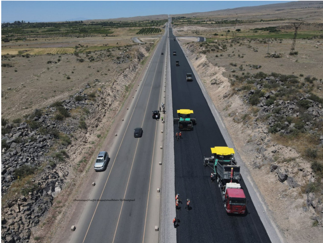
Figure 3. June 25, 2025 – km 48+000: Ongoing construction works for Task 2
