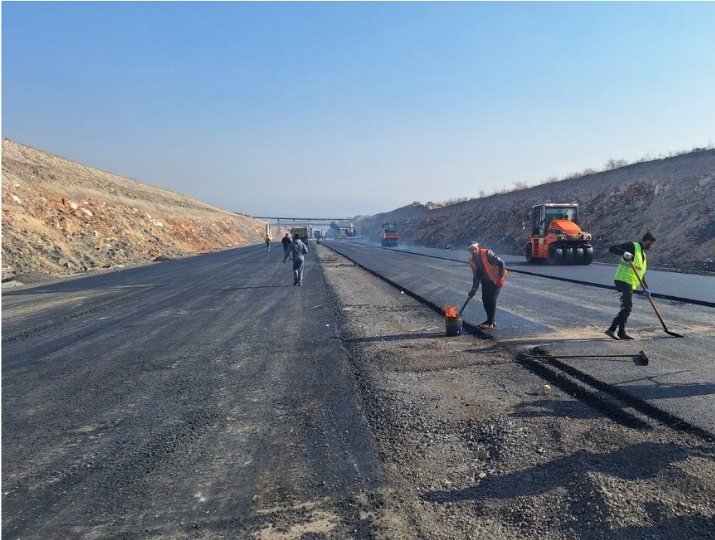
Figure 1. March 14, 2025 – km 35+700 – 35+900: Ongoing construction works for Task 1
